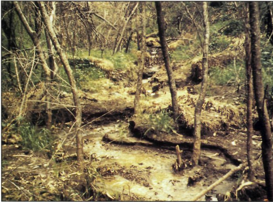
Photo 9. In March 1992, after an average rainfall season, 63 percent of all straw bale check dams in the North Oakland Sports Center watershed had failed.
