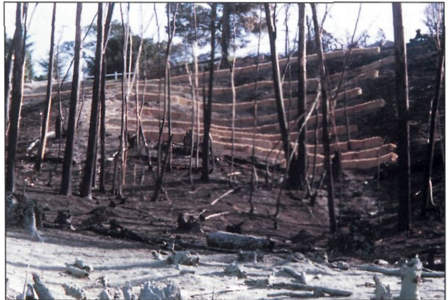
Photo 6. Straw bale check dams or dikes are paced in rows on an old landslide feature. In the foreground the hillside has been treated with the seed and hydromulch application which was eventually sprayed over the entire area.
