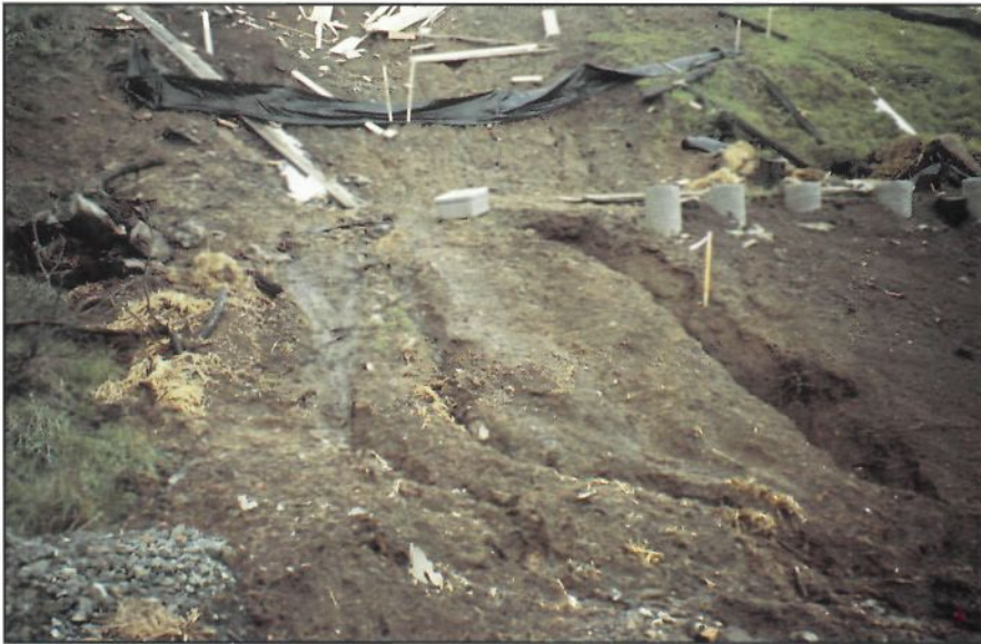
Photo 7. Construction initiated rilling and gulying. There was no erosion control at this site in the burn area.
