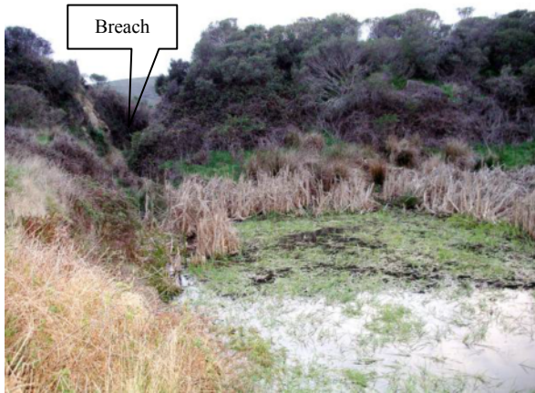
Figure 14: This photo shows the spillway breach in P-061 at the downstream end of the chain of impoundments along a tributary to Glenbrook Creek. A shallow, seasonal pool is retained in the excavation below the base elevation of the dam.
