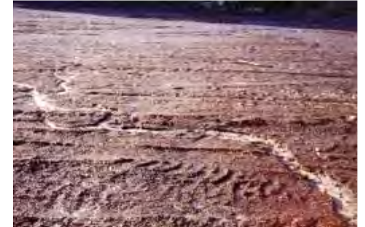
(Photo 21) An example of rill erosion in soils prepared for sod in Alvarado Park. Consider the amount of sediment production during preparation of the Tilden golf course during the late 1930s.
