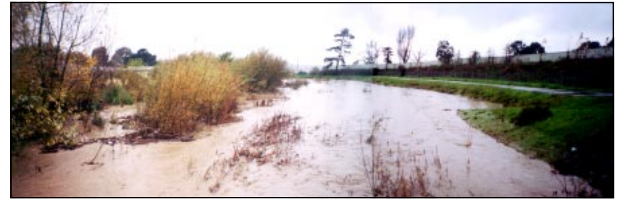
(Photo 54) The waning flood of January 1997 in the trapezoidal flood control channel divides between the constructed bankfull channel on the left and the constructed flood plain on the right. Debris has collected at the entrance of the low flow channel.
