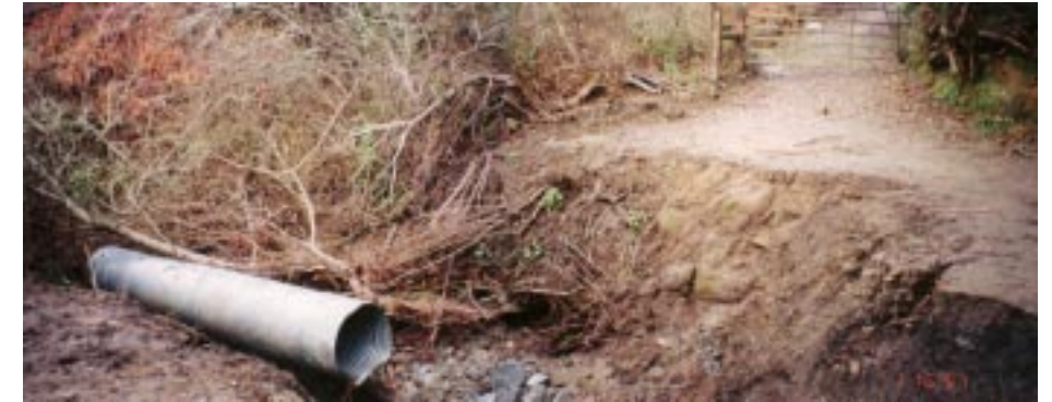
(Photo 4) A 3 ft diameter culvert fails along the Havey Creek Trail in the Lower Canyon Segment, January 1997.
