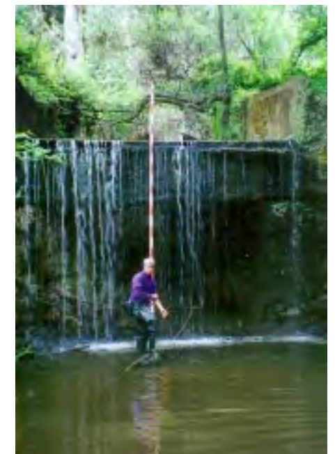
(Photo 36b) The edge of the spillway in 1999 has over 14 ft of fall.
