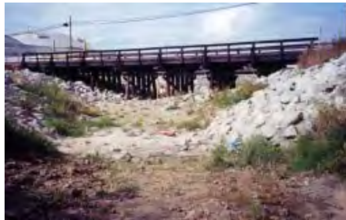
(Photo 29) Looking downstream at Santa Fe Railroad trestle and rip rapped trapezoidal banks of the flood control project, as represented in cross section "F" in Figure A (see facing page). The grouted rip rapped corresponds to the aggradation shown in Figure 89, page 69.
