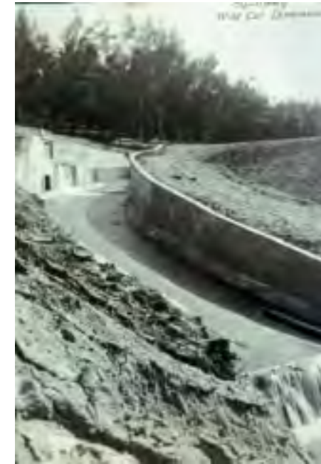
(Photo 36a) The edge of the newly constructed dam at Jewel Lake, 1922. Note there is about 2.5 ft of fall.
