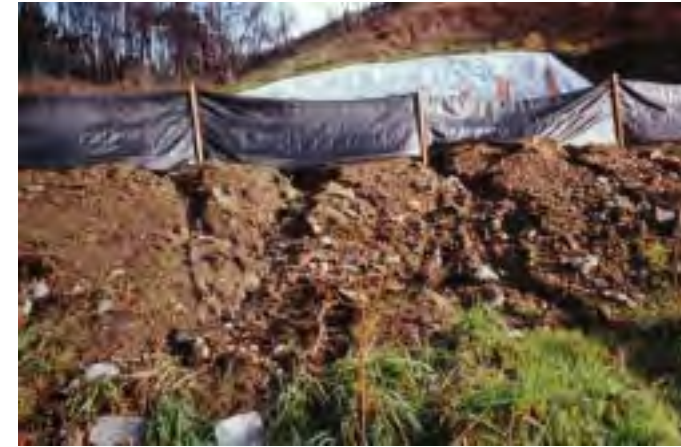
(Photo 20) Construction site erosion in disturbed soils. Soils that have been mechanically disturbed are more susceptible to erosion than soils that are bare but still have small rootlets intact. (Booker et al. 1993) Such a situation may occur after burning, grazing or application of herbicides.
